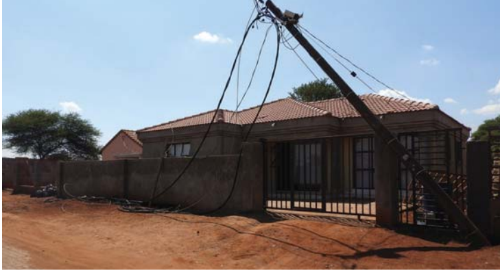
A truck reversed into an electricity pole, causing an explosion, leaving residents without electricity.
